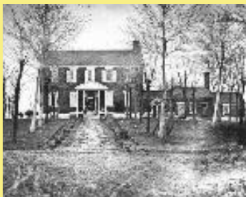
Historic view of Liberia House
